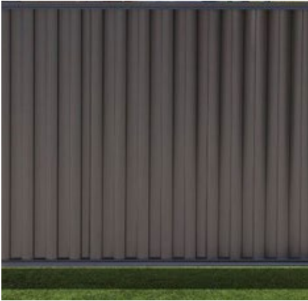
Side and Rear Fencing
