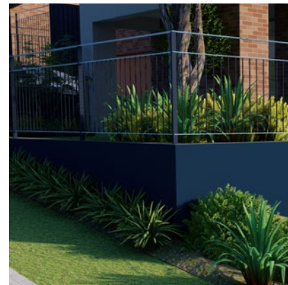
Rendered Masonry – Painted
